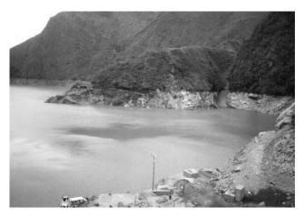
Figure 4. Rock and surficial sediment slides were potential danger to turbines.
