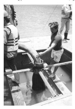
Figure 5. Filling of geotube in cradle.
