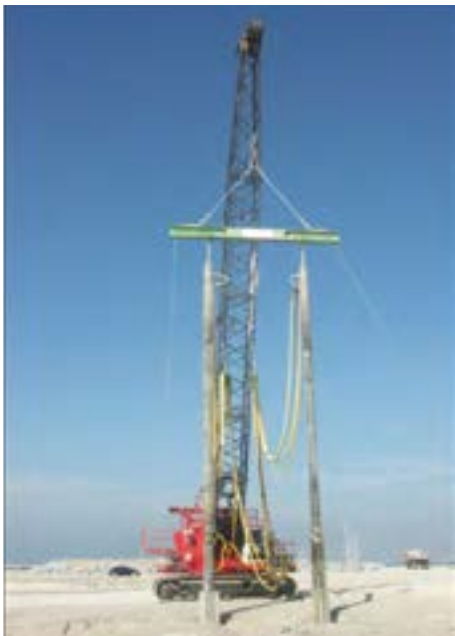
Sand Compaction
