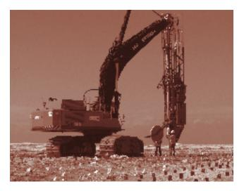
The wick drain system is one method used to hasten the removal of water from soil. Here, wick anchor plates are being used to mark the location of each wick prior to installation.
