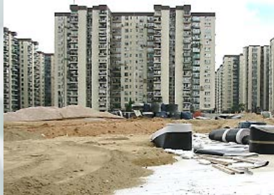
Deckdrain at Mei Foo Station during installation
