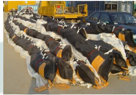
Standard packaging of prefabricated silt curtain at Kai Tak development
