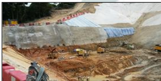
GFRP anchors, installed at the portal
