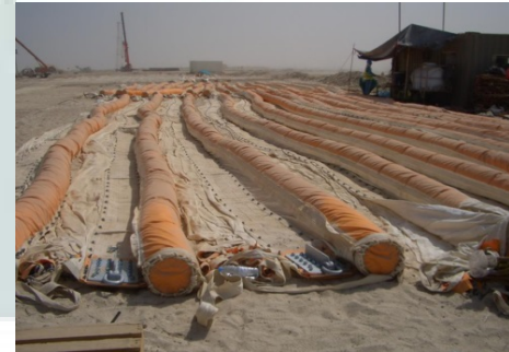
Engineering designed silt curtain from Japan at Penny's Bay
