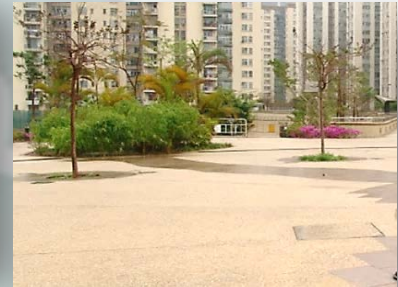
Mei Foo Park Deckdrain drainage
