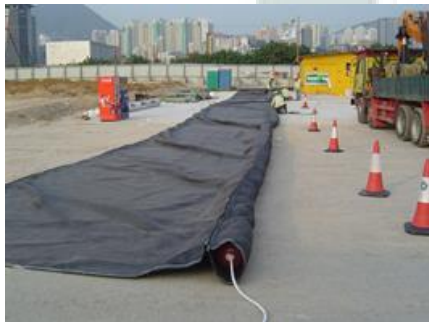
In-situ silt curtain fabrication from Bontec geotextile, limited reinforcement
