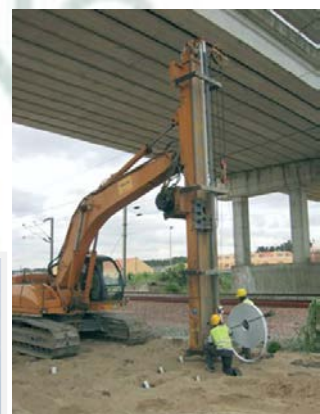
Telescopic mandrel with 8m headroom to great depth
