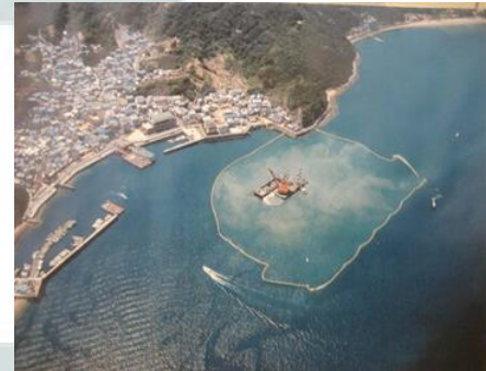
Turbidity control of engineered silt curtain
