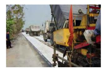
Pavement fabrics go a long way in extending the life of your pavement. There are fabrics designed to help stabilize sub-soils and prevent ground contamination, fabrics to help water filter under pavements and overlay fabrics to retard reflective cracking.
