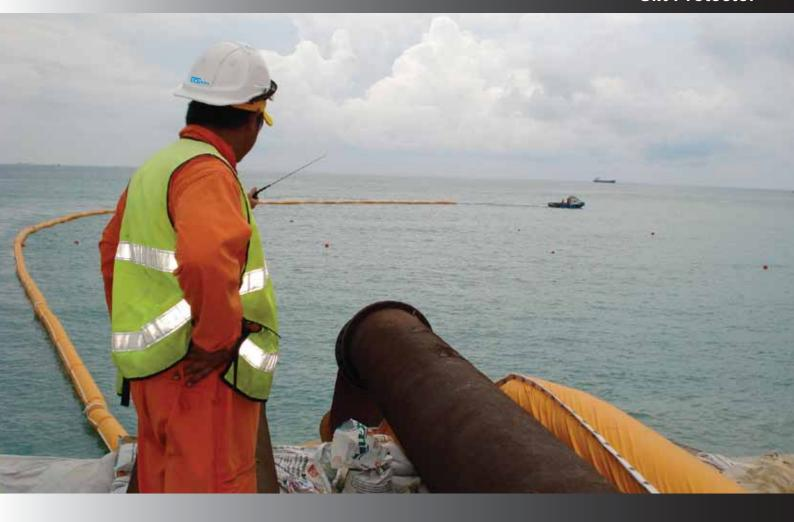
A Silt Protector is a flexible membrane product consisting of woven geotextile that has been designed to physically prevent diffusion of pollution generated in dredging or reclamation works on the seas or rivers.
