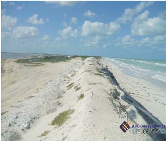
Photo 1 Geotextile Back Beach Protection.
