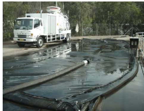
Photo 9 Filling of geotextile tube commences
