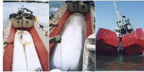
Photo 5 Geotextile Container in Barge
