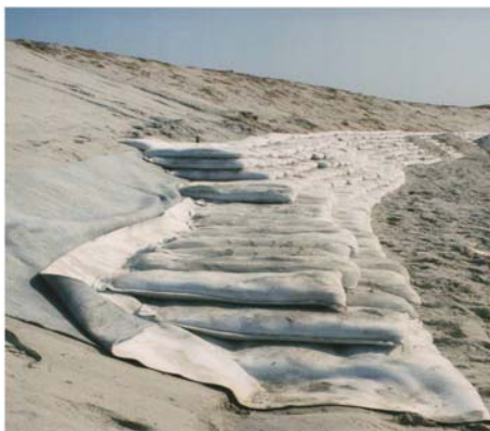
Photo 6 Geotextile Bag Placement.
