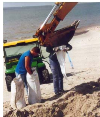
Photo 7 Filling Geotextile Bag
