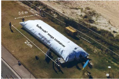
Photo 4 Geotextile Container
