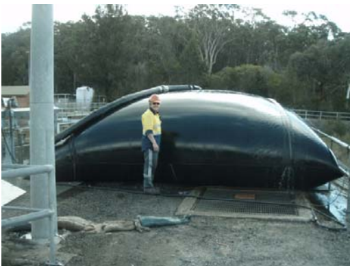
Photo 10 Geotextile tube filled
