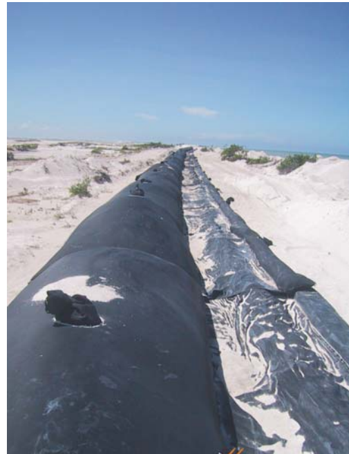
Photo 3 Geotextile with Scour Apron
