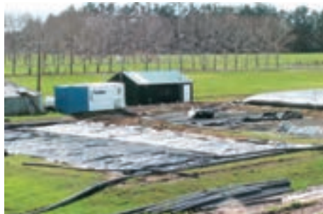
CeTeau Tube Placing
