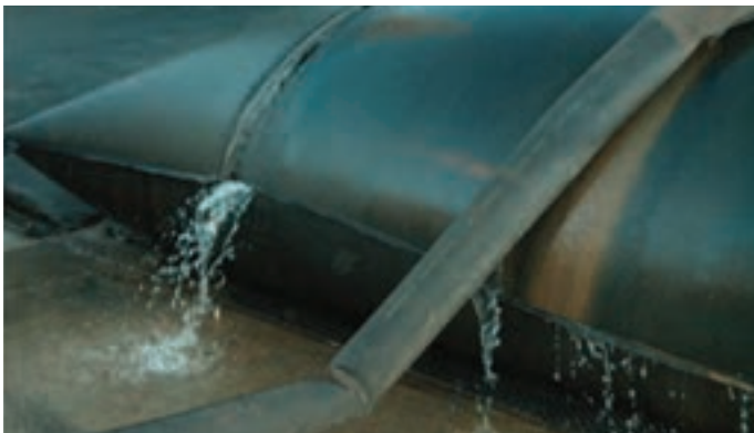
CeTeau Tube Dewatering
