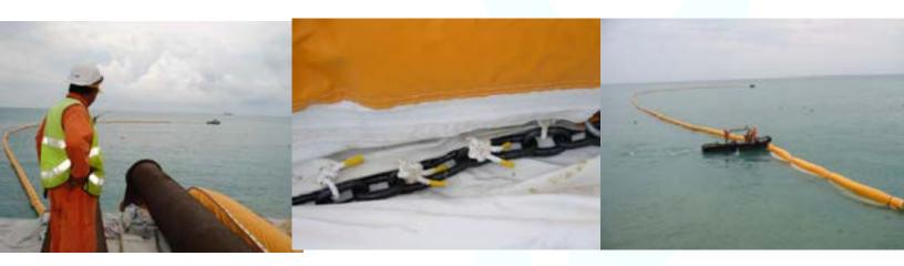
A Silt Protector is a flexible membrane product consisting of woven geotextile that has been designed to physically prevent diffusion of pollution generated in dredging or reclamation works on the seas or rivers.
